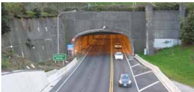
The southern portal entrance to the Terrace Tunnel, Wellington. Completed in 1977, it was originally designed to have a twin. As a Road of National Significance the original plan will now be realised.
