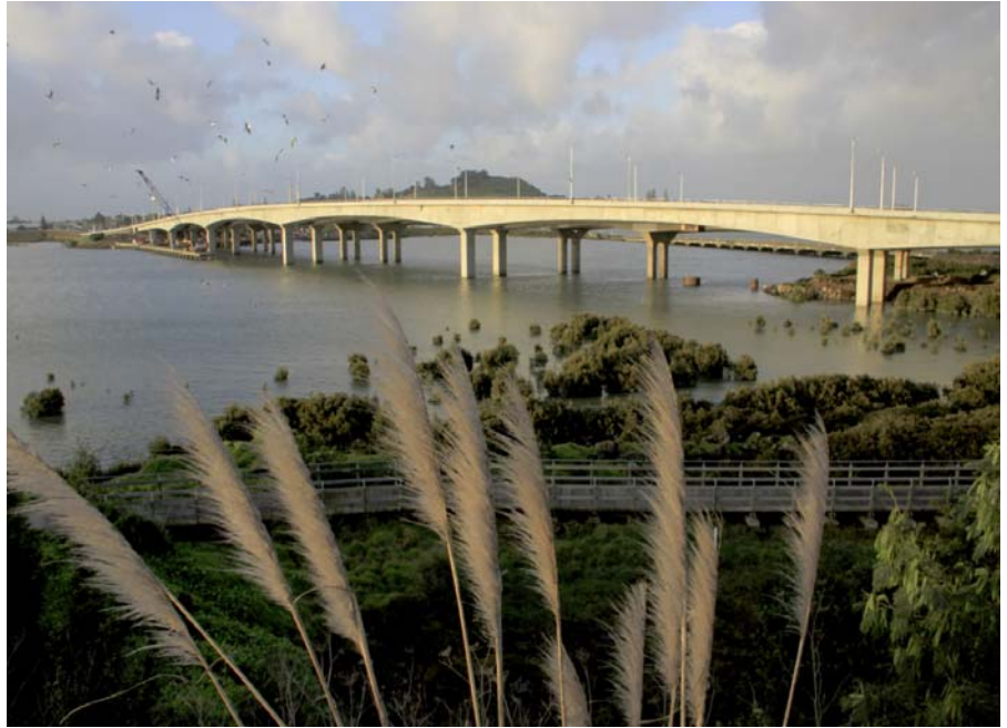
Mangere Bridge. MHX improved public transport connectivity by providing bus shoulder lanes and provisioned for a future rail link along the route. Three and
