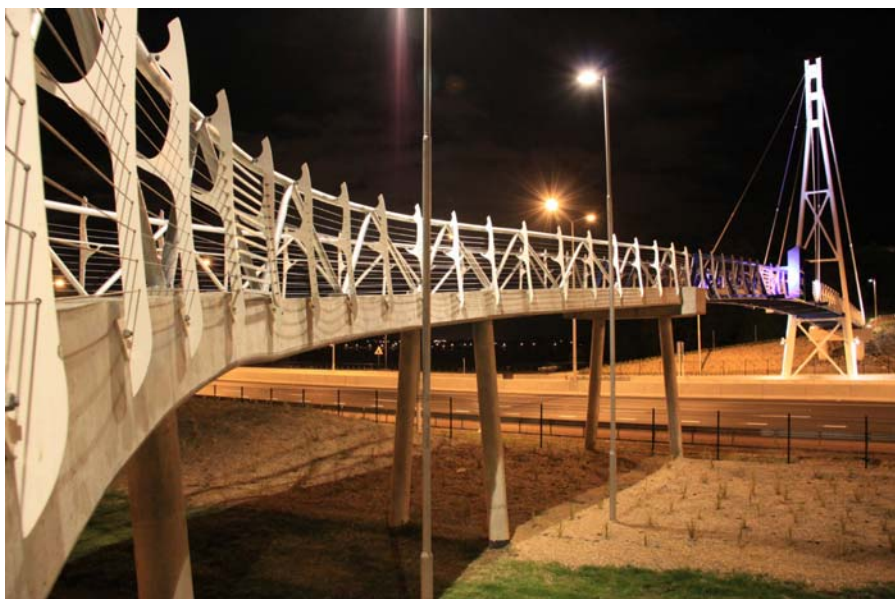
BELOW: The Beachcroft Footbridge.
